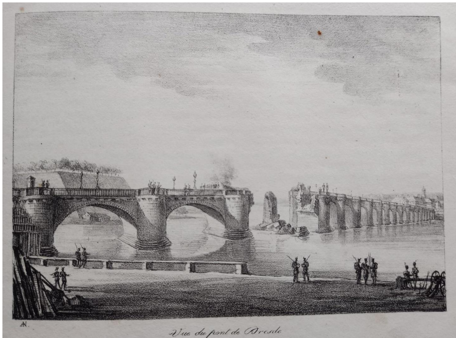
View of the bridge at Dresden in May 1813 – from item 65
