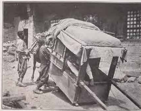
THE MOUNTAIN LITTER, Putting in the hind mule.
